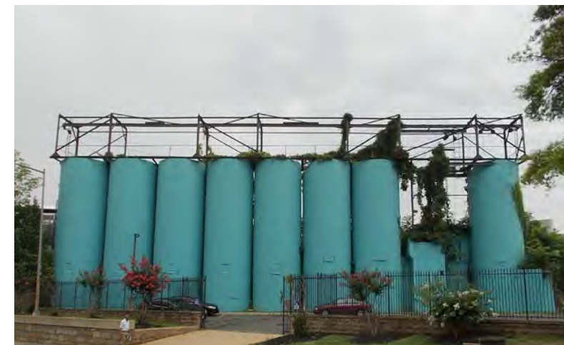
J. Silos on Rhode Island Ave.
