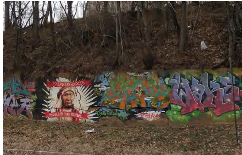
E. Retaining wall
