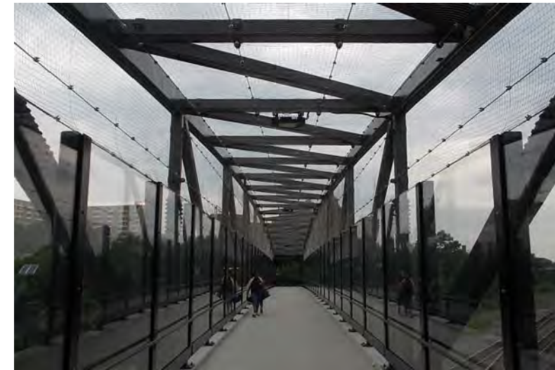
F. Metro Bridge
