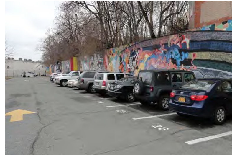
F. Retaining wall
